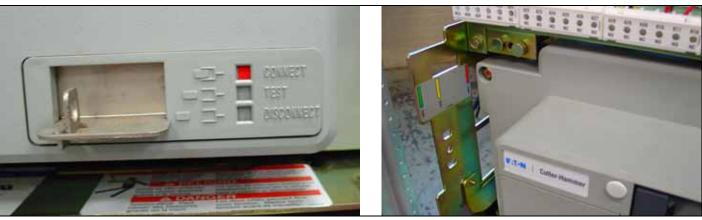
Figure 29. Switching Device in the CONNECT Position.
